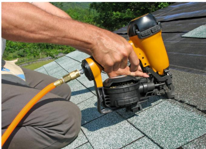
4. Continue installing shingles in the same fashion along the eave. The shingle ends just butt into each other.
